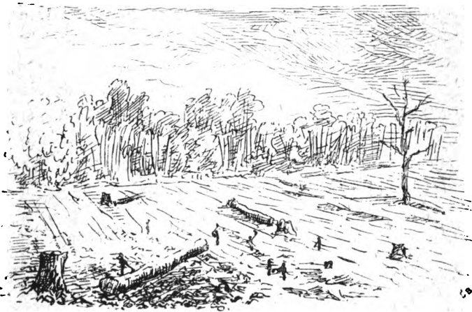
CLEARING THE GROUND.
